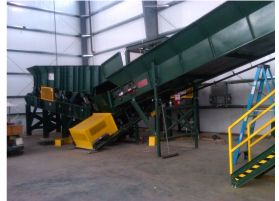
Construction debris starts at this end of the conveyor
